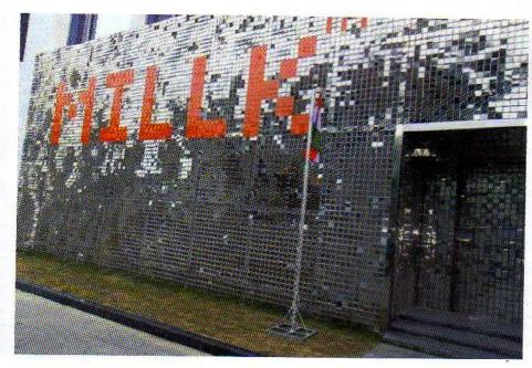
This dynamic façade in Mumbai is designed with thousands of metal sheets suspended with pin joints. The air movement over the surface is mimicked by the metal panels creating patterns and multiple reflections as per the intensity of the wind on it. The concept is very similar to the Technorama science center, the only difference is its much smaller scale and the effect is limited to a smaller area than desirable.
